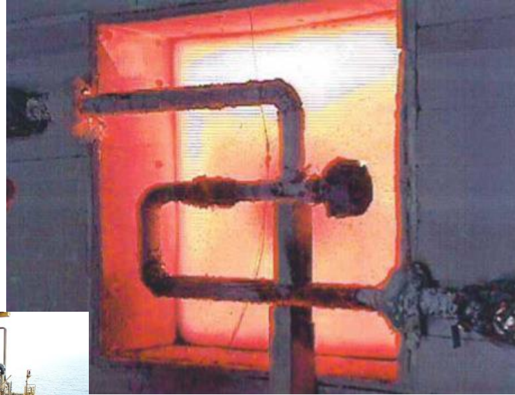
Future Pipe Industries
