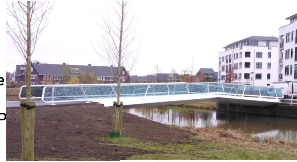
'Bronlibelle' Bridge in Harderwijk, the Netherlands. A 6.3 m wide, 22 m long GFRP bicycle / footbridge connecting two new districts of Harderwijk.
