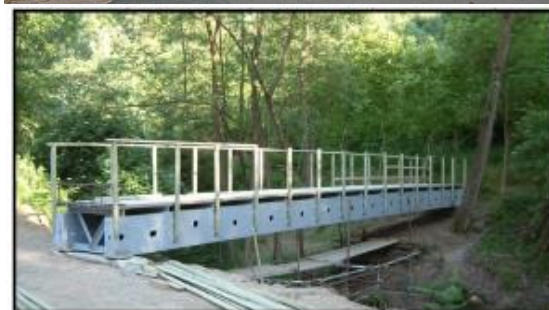
Pultruded GFRPs, Italy, pedestrian bridge, 2004.
