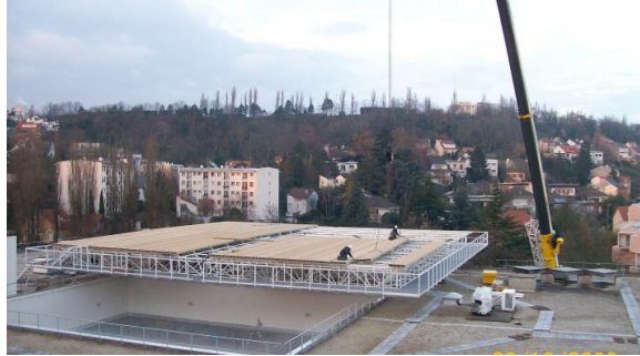
Plessis Robinson (92) France. Helipad made with pultruded GFRP profiles
