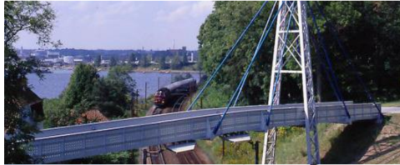
Kolding, Denmark. Pedestrian and cycle bridge from 100% pultruded GFRP profile, 1992
